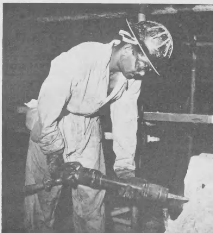
A SAFETY lens in P. J. Cicilia's chopper goggles was shattered when a piece of concrete struck it with bullet-like force while the Mechanical-Yard employee was chipping concrete at No. 2 Powerhouse. Fortunately the lens of the safety goggles was destroyed and not his right eye which once again demonstrates the impact resistance of safety lenses.
